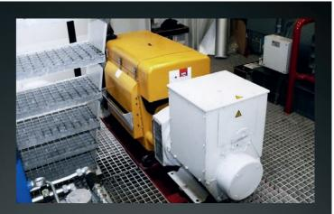
The compact systems can be installed easily and within the smallest space: on the one hand because of the engines' air cooling and, thus, the prevention of a front end cooler or an interface with the ship-based cooling system. On the other hand through the use of liquid cooled turbo diesel engines of the new Hatz H-series and their extremely compact installation dimensions.
